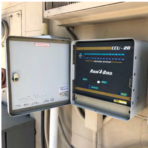
Inside a CCU Enclosure
